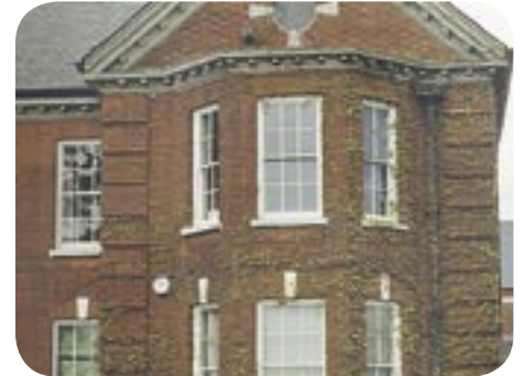
Front bay of main administration building
